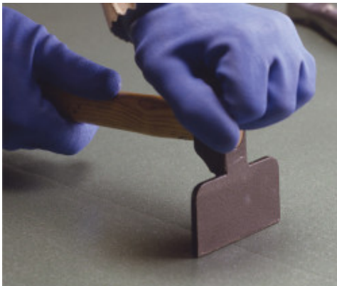
Pressing down the junction between sheets
