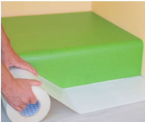
1. Placement of Mapecontact Plus on the tread and then on the riser
