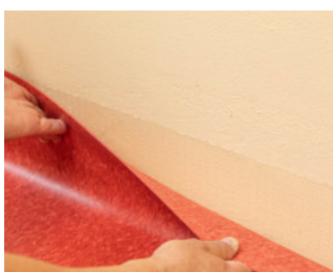
7. Installation of the coving on the wall
