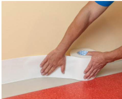
1. Placement of Mapecontact Plus on the wall
