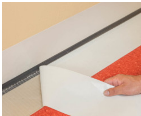
5. Removal of the protective layer from the floor
