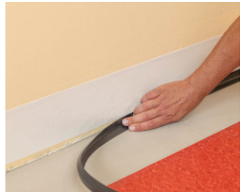
3. Installation of the cove former
